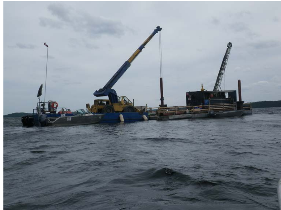
Diamond Drill Rig (Barge)
